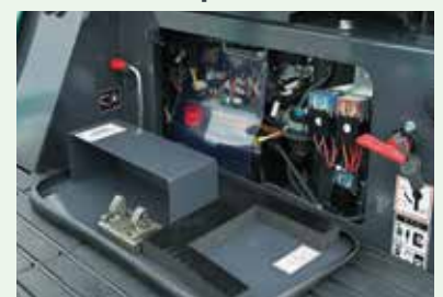
•Generator •Starter motor
